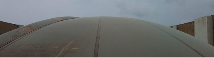
Gas capture balloon over Combiteat unit
