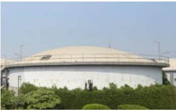
Sludge digester
